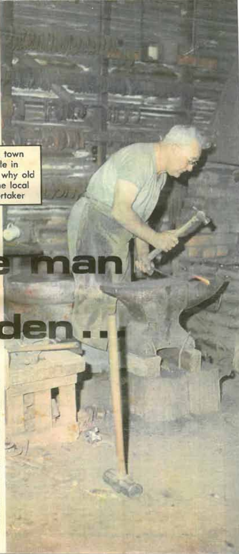
★ RIGHT: Craftsmen at work — the master Bill Roberts assisted by apprentice Anthony Ryan turns red hot metal into a horseshoe.
