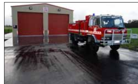
The new Jancourt Fire Station, officially opened on June 17 th .
