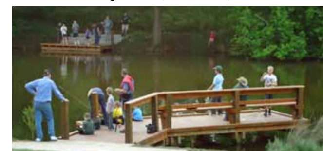
Two of the five new jetties on Lake Cobden officially opened on October 14 th by Hon Terry Mulder MLA
